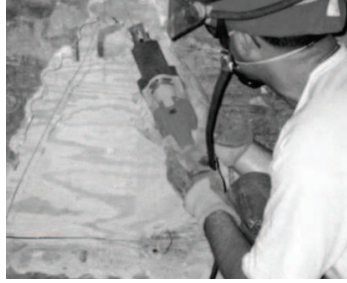
Figure 6 ▲ Cutting a wood panel
