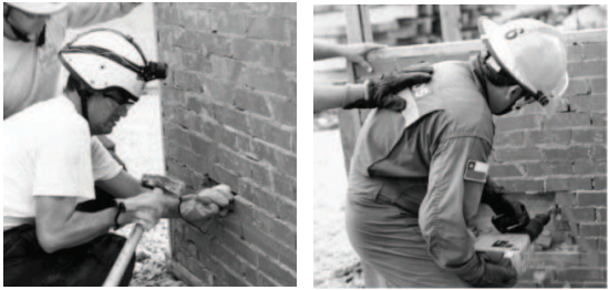
Figure 8 ► Breaching a brick wall
